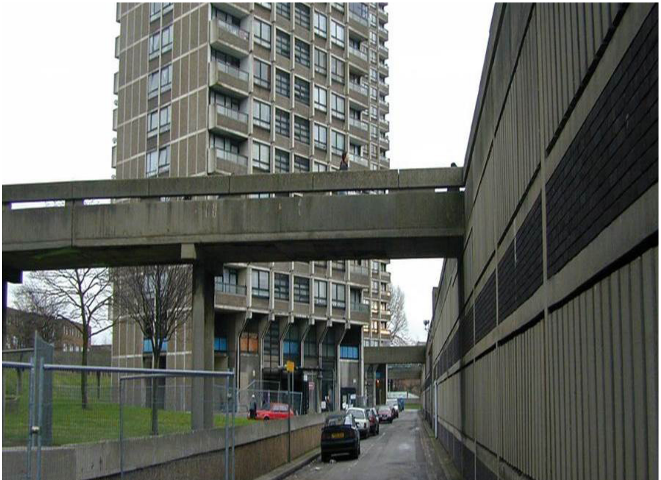
CROSSWAYS ESTATE BEFORE EXTENSIVE REFURBISHMENT, TOWER HAMLETS
