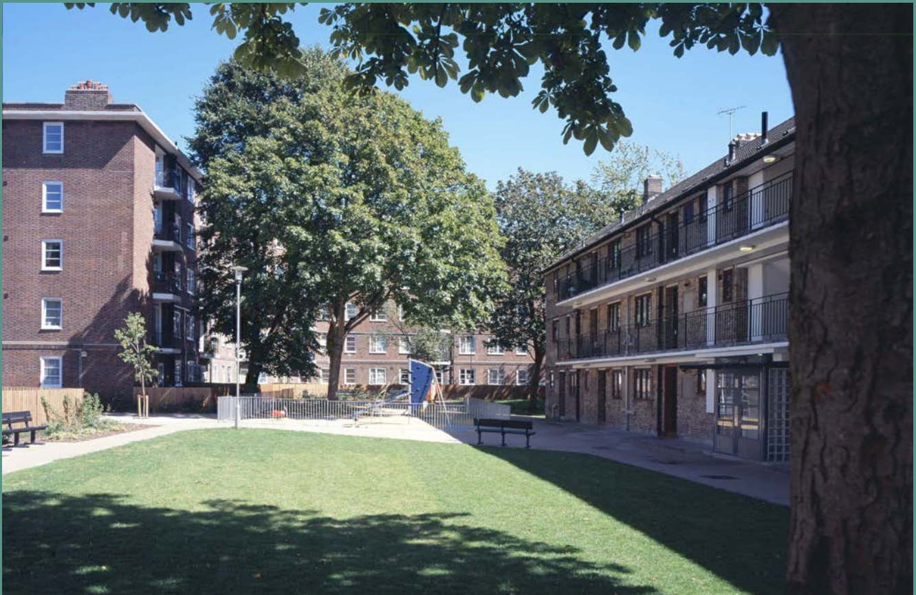
CLAPTON COMMUNITY CONSORTIUM, HACKNEY - REFURBISHMENT OF POPULAR OLDER STOCK
