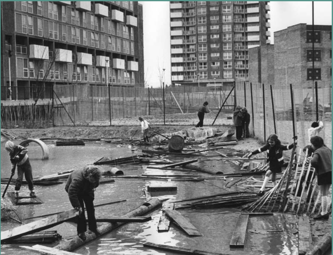
CATHALL ROAD ESTATE, WALTHAM FOREST BEFORE REGENERATION (MUSEUM OF LONDON)
